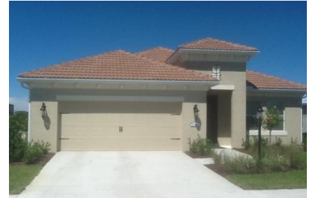
Gutters on Front Elevation
